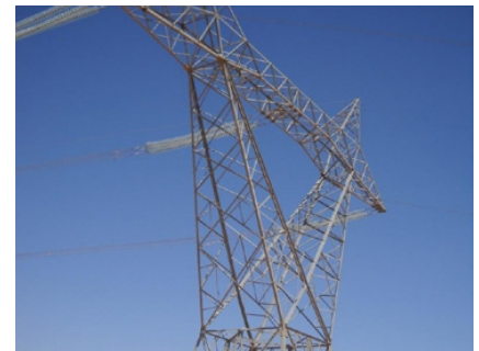
GECOL - LIBYA, Turn-key 400kV TL
