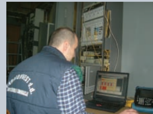
SDH&DWDM Transmission Systems
